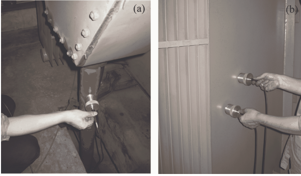
Fig. 6. Collection of PDs from a field transformer. (a) The sensor is attached to the cable insulation, (b) The sensors are attached on the metal tank wall.
